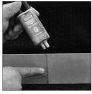
Apply sandable epoxy (P/N ACA-SCF) to face of joint, let set and sand flush. Mud & finish bottom of light cove as required then primer and paint.
