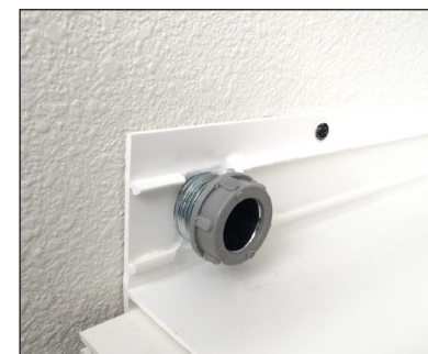
Figure 4 Determine where the start of the runs will be and drill a hole for the conduit feed in between runs.
