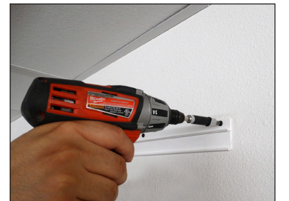
Figure 3 Secure the mounting rail to the wall using the supplied wall-dog screws.
