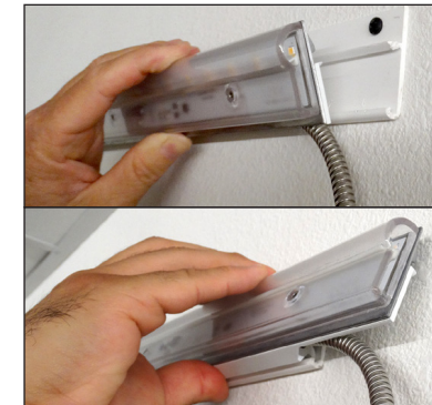
Figure 8 Attach pr1meFX by placing the bottom side over the bottom lip of the rail and then carefully pushing the top of the fixture onto the rail until it snaps into place.
