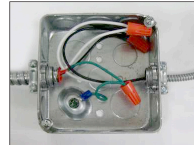
Figure 1 Connect field wires to the pr1meFX power feed cable(s) inside the grounded J-Box.
